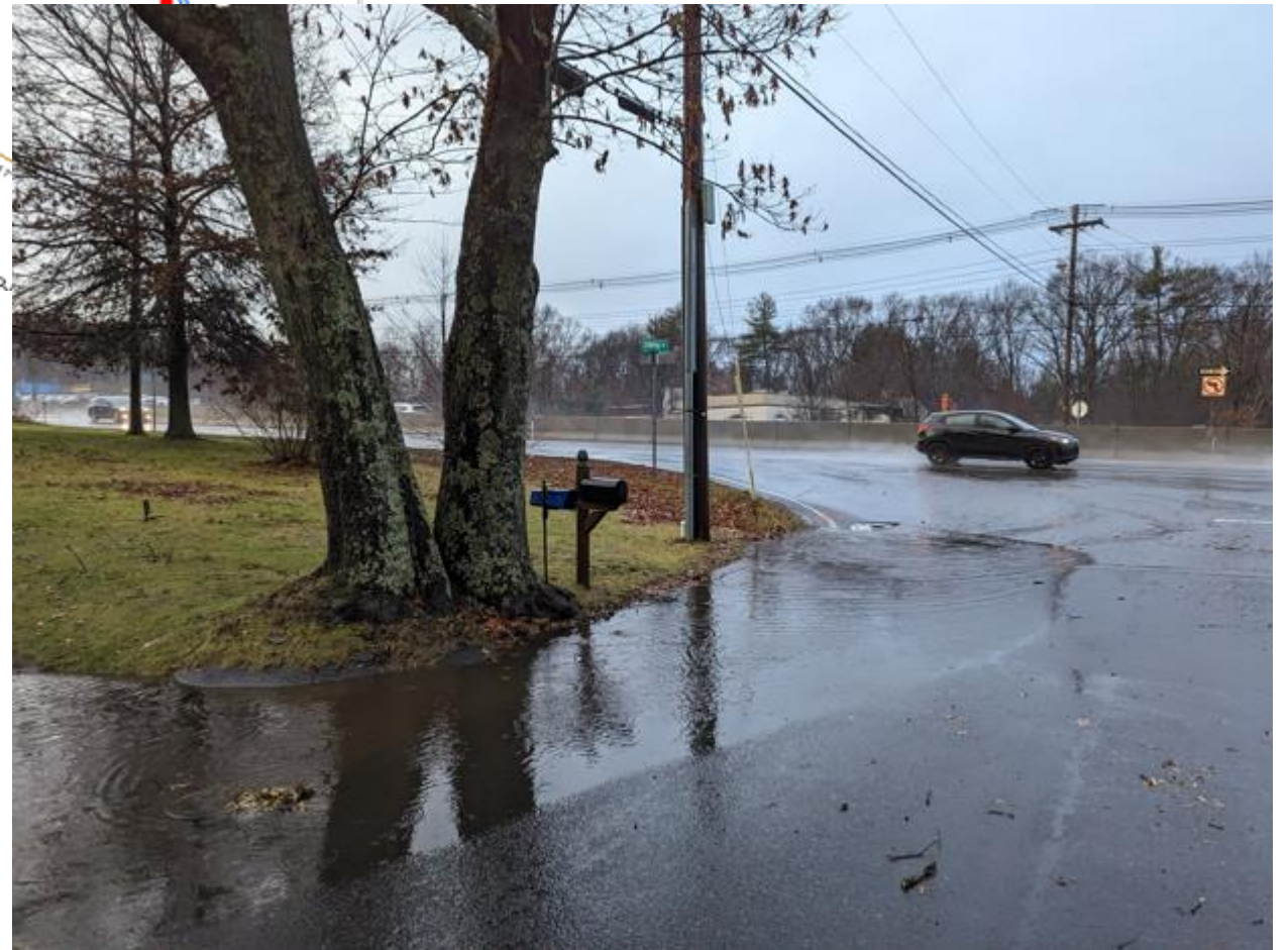
Typical flooding at Route 9 & Parkerville South Side Intersection
