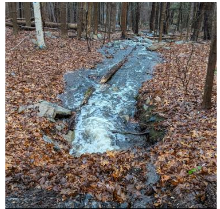
Other side of Parkerville at the Parkerville culvert
